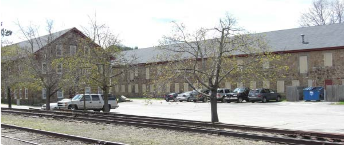
Existing Conditions Store House (left) and Long Shop (right)
