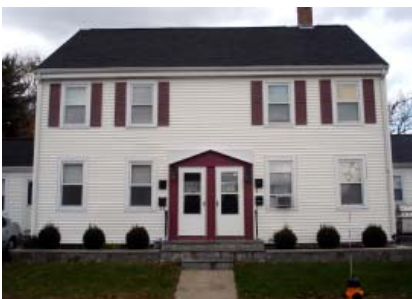
Worker's Housing (Reused Sections from the Original Wood Factory Buildings)
