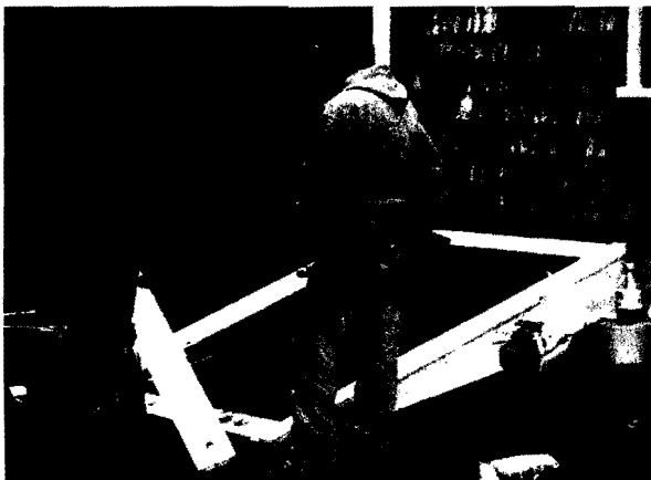
A new bulkhead for the Harlow Farmhouse Ellisville Harbor State Park, Plymouth
